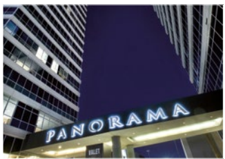
Panorama Towers 137 MOBOTIX Cameras, U.S.A.
