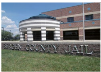
Bergen County Jail 820 MOBOTIX Cameras, U.S.A.
