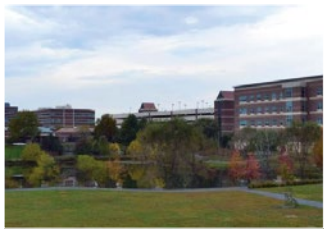
Valley Health Hospital 100+ MOBOTIX Cameras, U.S.A.
